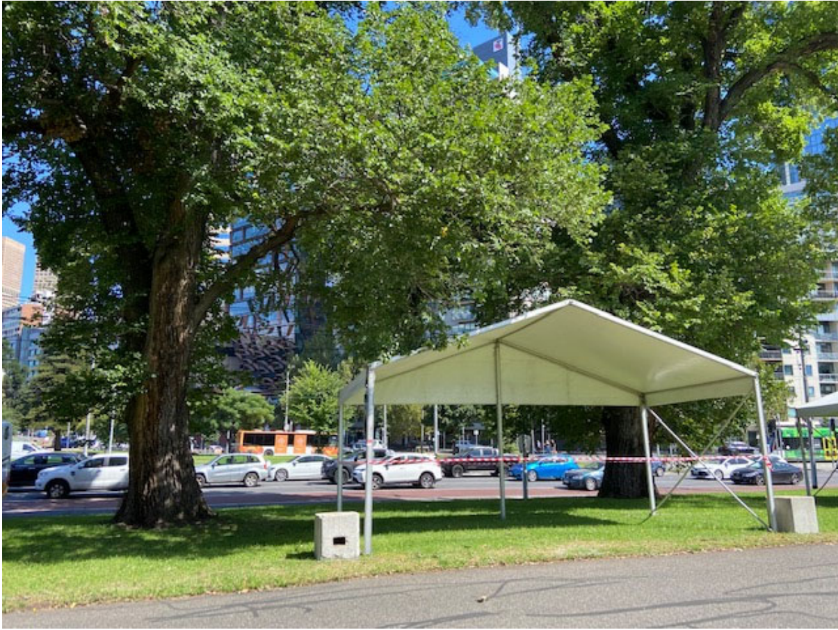
Setting up with concrete blocks directly underneath the canopy of trees. No matting.
